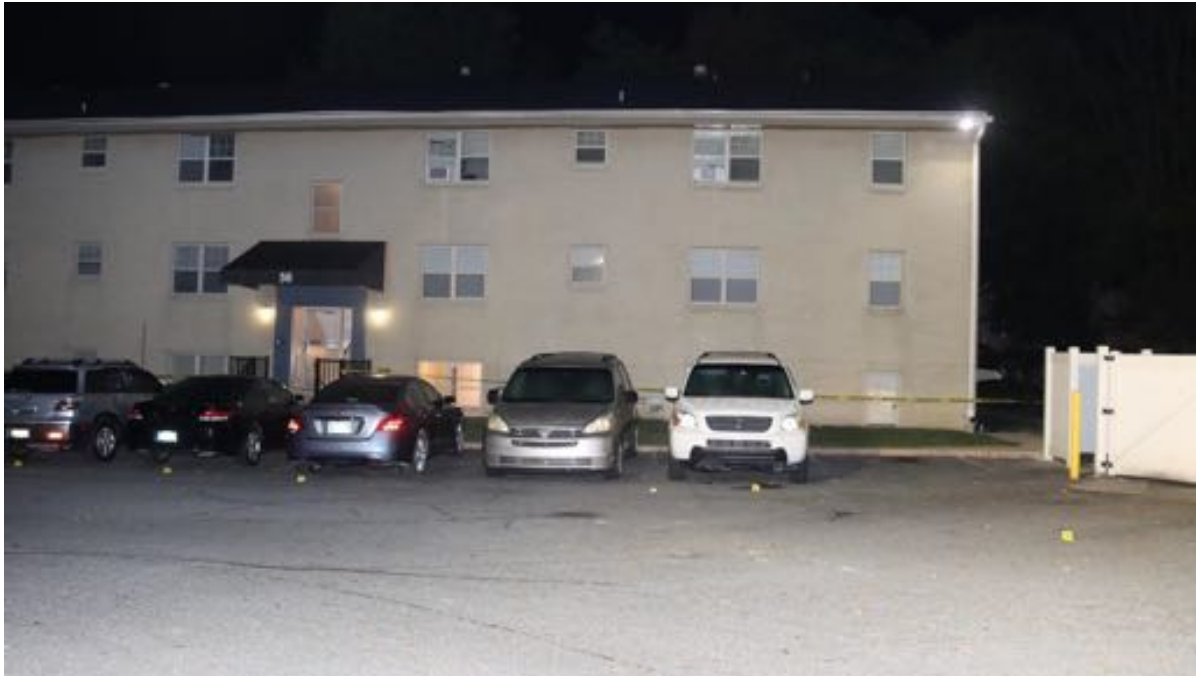
Four personal vehicles that were struck by gunfire. The building's brick facade and the plastic dumpster enclosure also sustained projectile strikes.
