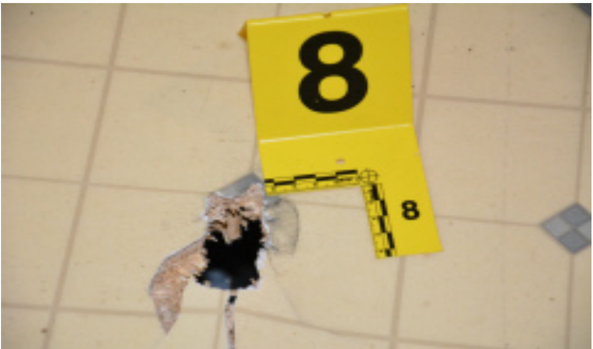
Damage to the floor caused by the shotgun round.
